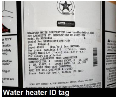
Water heater ID tag
